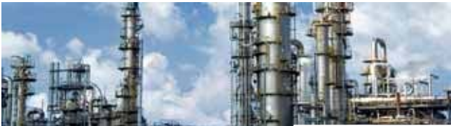
PETROL-CHEMICAL REFINERY PLANTS
