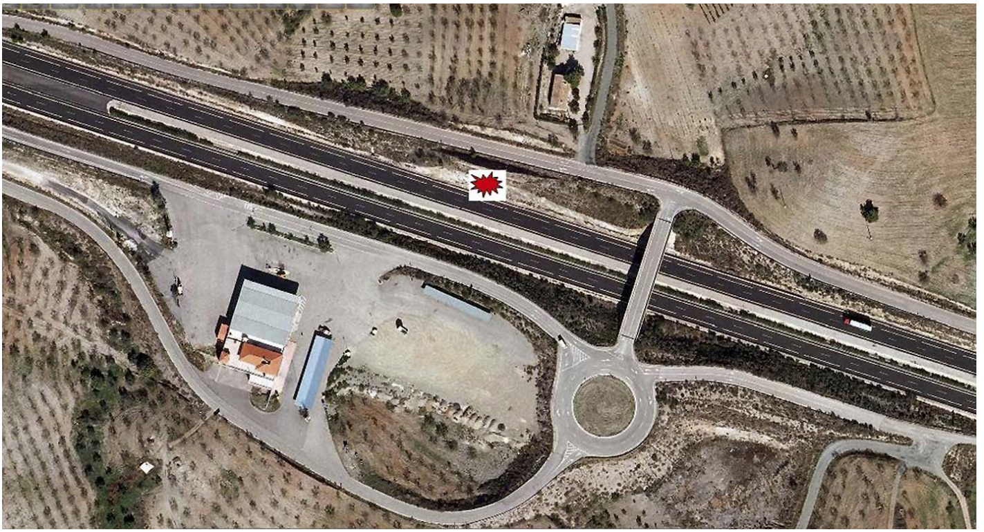
Figure 1. Bird's eye view of the accident area. Source (1)
