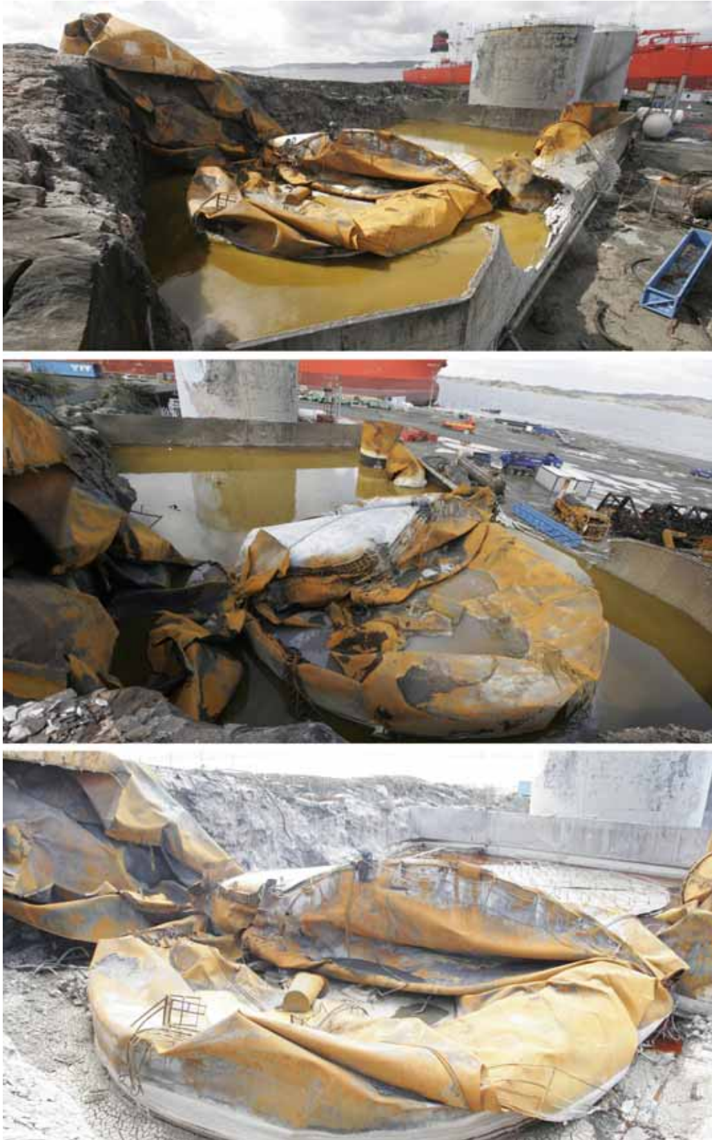
Figure 3-3 Various pictures of Tank farm II viewed from the north, illustrating the damage to the 5 tanks, the bund, the office building, the two tank lorries, and the vacuum truck; pictures from The Norwegian Police, taken 25 th May 2007 (above and centre) and 31 st May 2007 (below).
