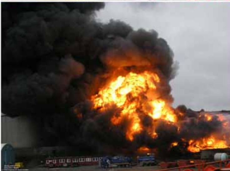
Figure 1-5 A series of pictures taken from M/T Karen Knutsen that illustrates how the fire in Tank Farm II developed during the first minutes after the first explosion in tank T3 on 24 th May 2007. Photographs provided by Glenn Rogers, Chief Engineer, M/T Karen Knutsen.
