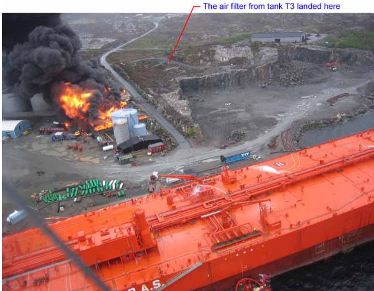
Figure 1-4 Picture taken from a helicopter from Norsk Luftambulans (Norwegian Air Ambulance) about 45 minutes after the first explosion, showing the tanker M/T Karen Knutsen, most of the tank facility, and the extensive fire in Tank Farm II. The fire in the red office building has started, presumably due to radiative heat transfer from the fire in the tank farm. The picture also shows where the air filter from tank T3 landed, as well as various details not included in Figure 1-2. Photograph provided by Lasse Fossedal from Norsk Luftambulans.
