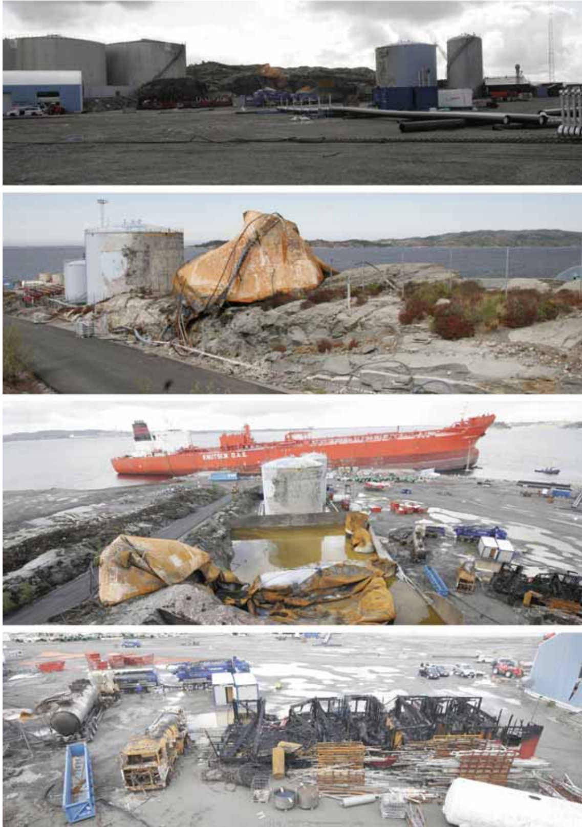
Figure 1-6 Overview pictures illustrating the tank facility at Sløvåg after the accident on 24 th Mai 2007: Tank farm II viewed from the quay (25 th May 2007); the remains of tank T3 viewed from the road (26 th May 2007); Tank farm II with Tank farm I and M/T Karen Knutsen in the background (25 th May 2007); damages to the trucks and the red office building (25 th May 2007); photographs from the Norwegian Police.
